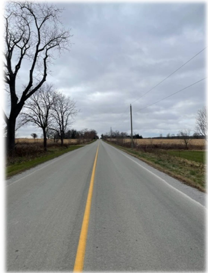
2023 Capital Project: Langan Drive Resurfacing
